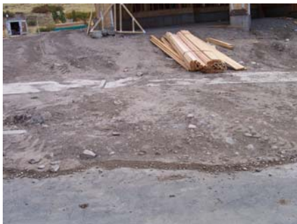
It is not uncommon to find massive amounts of dirt in gutters at construction sites
