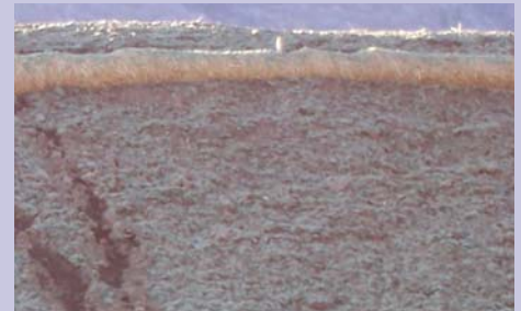
This slope has been hydro-seeded to encourage quick re-vegetation
