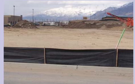
Silt fence is designed to stop dirt from leaving construction sites
