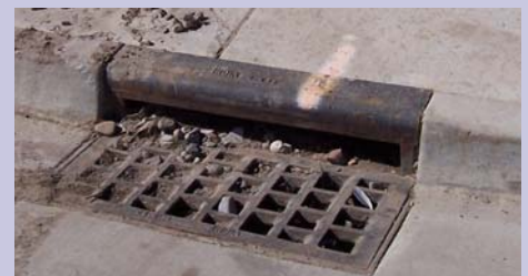
Improper erosion prevention and sediment control can damage storm drains and potentially cause flooding
