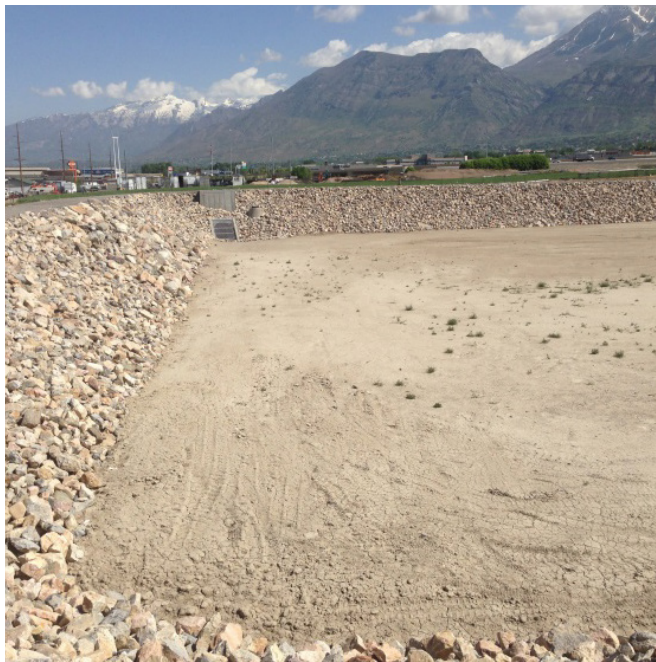
Williams Farm Detention Pond
